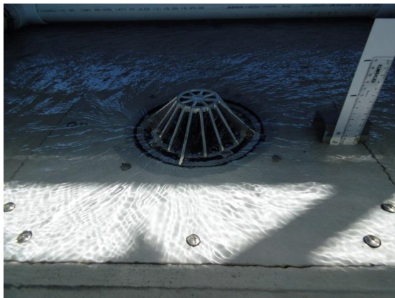
Weir Flow – 8 L/s (30mm)
